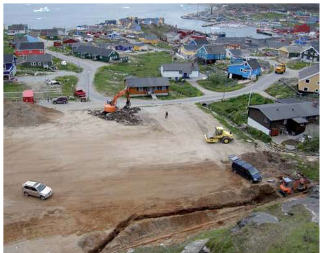
Figure 6: sub-base preparation for a FIFA Goal project in Greenland
