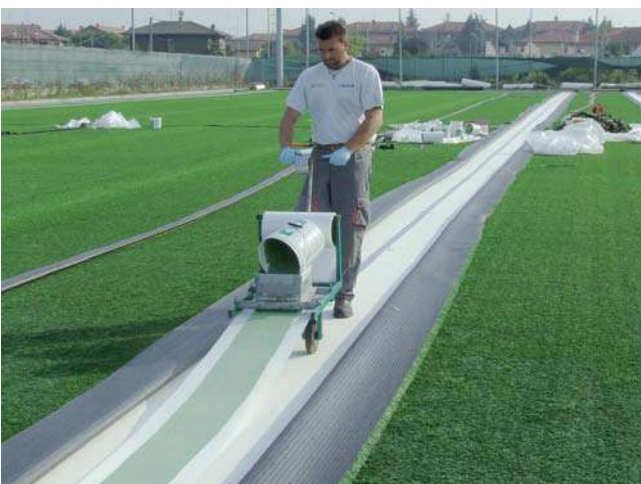
Figure 8: preparation of the seam tape
