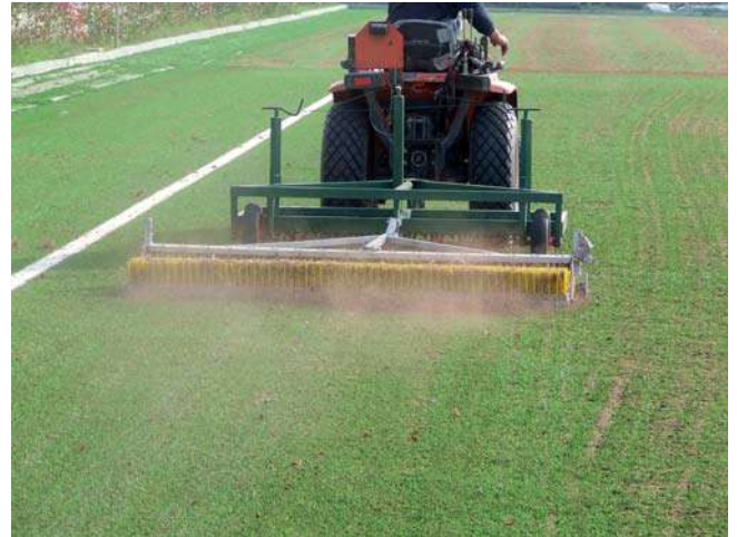
Figure 9: installation of the infill material
