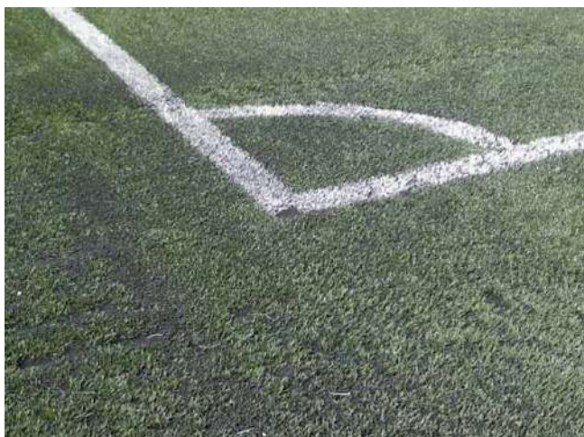
Figure 14: accumulated infill material in the corner area
