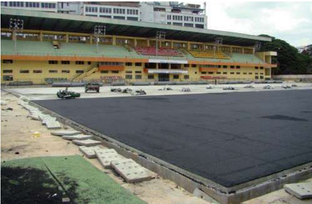
Figure 7: installation of an e-layer
